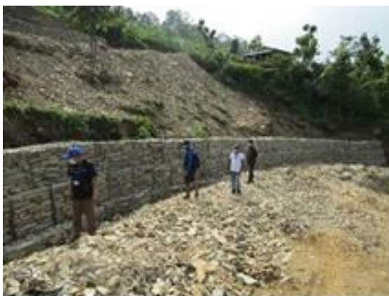
Figure 3: Gabion wall construction at Bodiswanra as landslide mitigation
