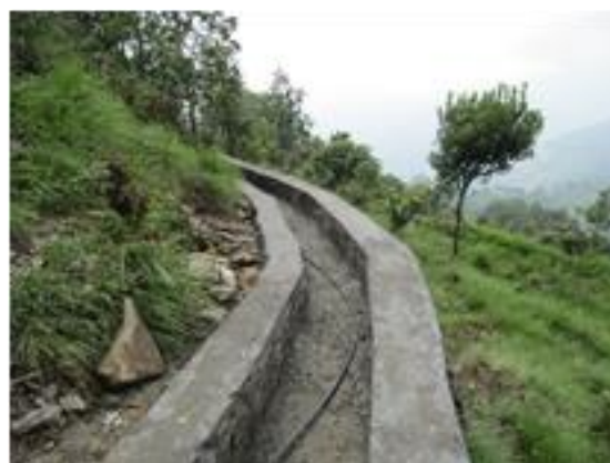
Figure 4: Water drain construction at Mathillopam so that the rain water drains through this and seepage and landslide can be minimized
