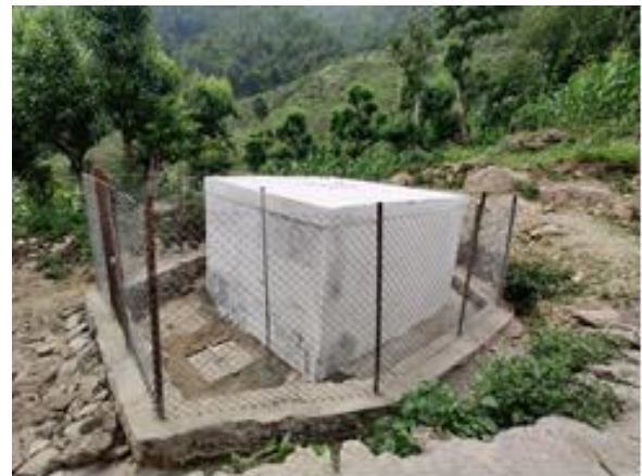
Figure 6: Drinking water system repaired through Rectification and construction of sectional Valve chamber at Chilaune scheme
