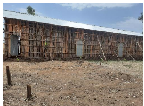
Figure 28: Classroom built by CSC at Kidist Hana kebele, Fogera woreda.
