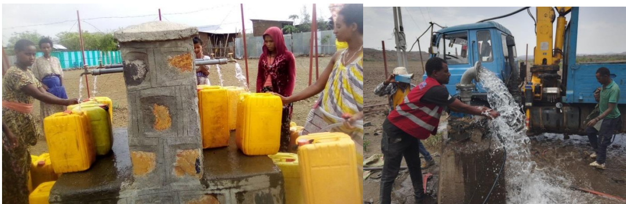
Figure 4: Community fetching water from solarized water schemes in Guhala; and pump testing after the installation of solar-powered water schemes
