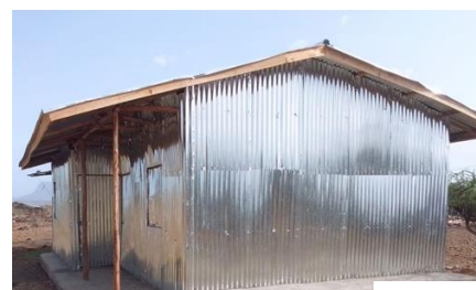
Figure 8: Kalay kebele Karita Wuha watershed users cooperative office, W/Belessa
